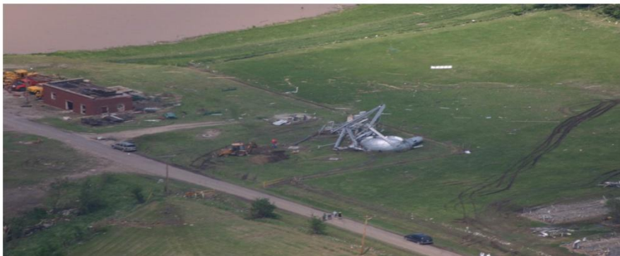
Jewell City Water Tower
